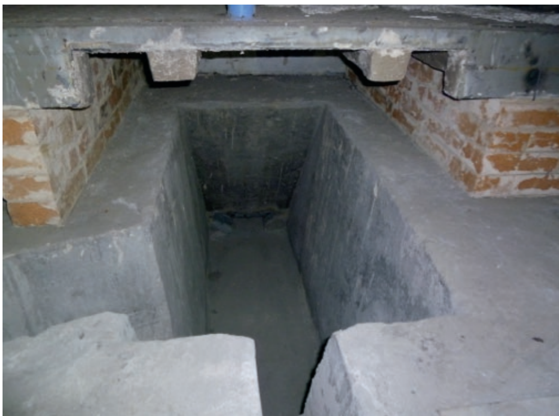
Launder of cupola furnace
