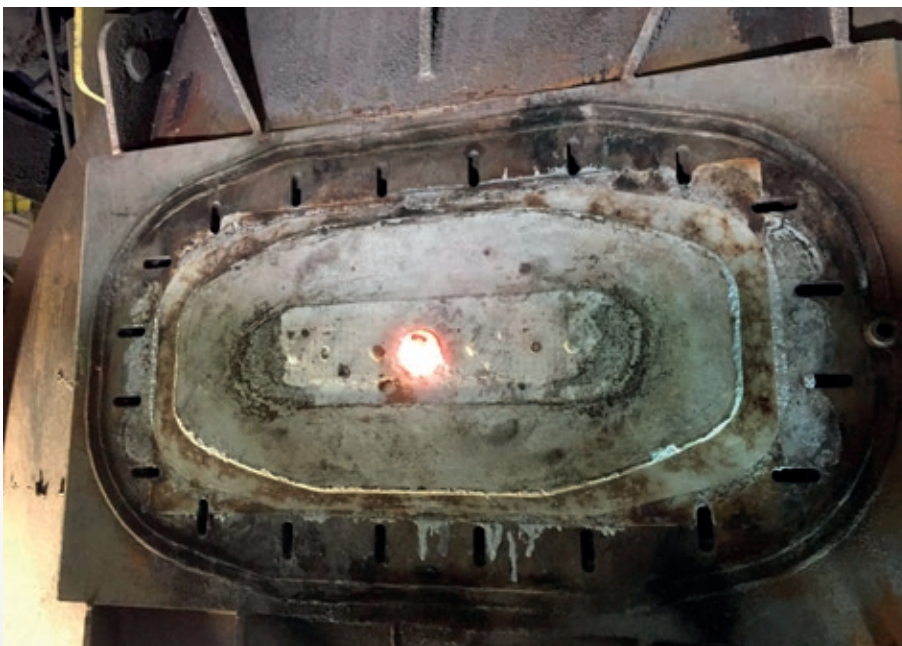
Installation of channel inductor
