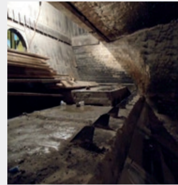
Partial re-lining of a grate combustion chamber.
