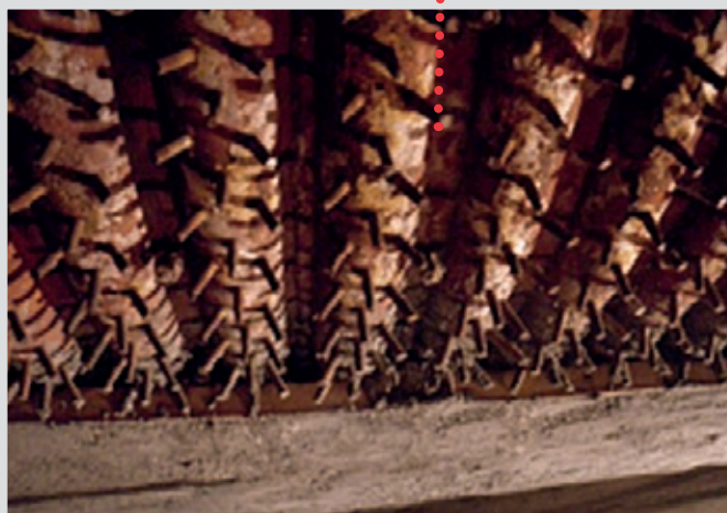
Lining by gunning of a membrane wall roof in an incinerator
