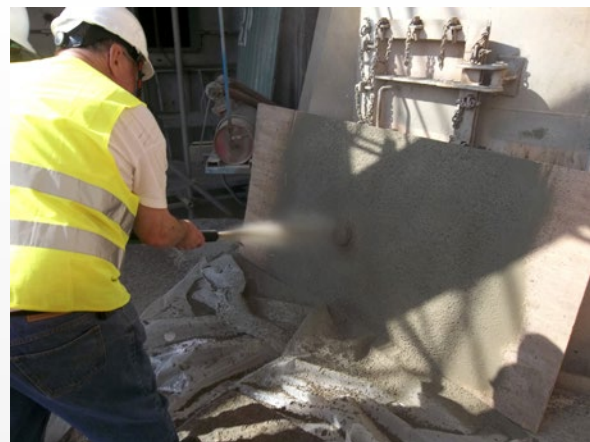
Gunning installation Tuning of the gunning machine
