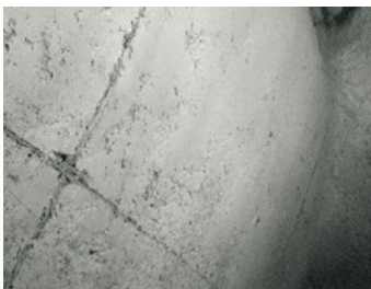
Smoke chamber. Low cement gunning application
