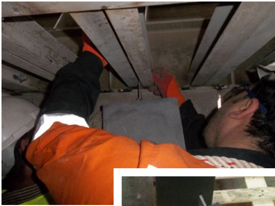
Precast Shapes: Grate cooler roof application
