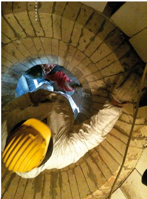
Cyclone – Bricks installation.
