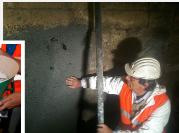
Shot Creting installation. Quality inspection
